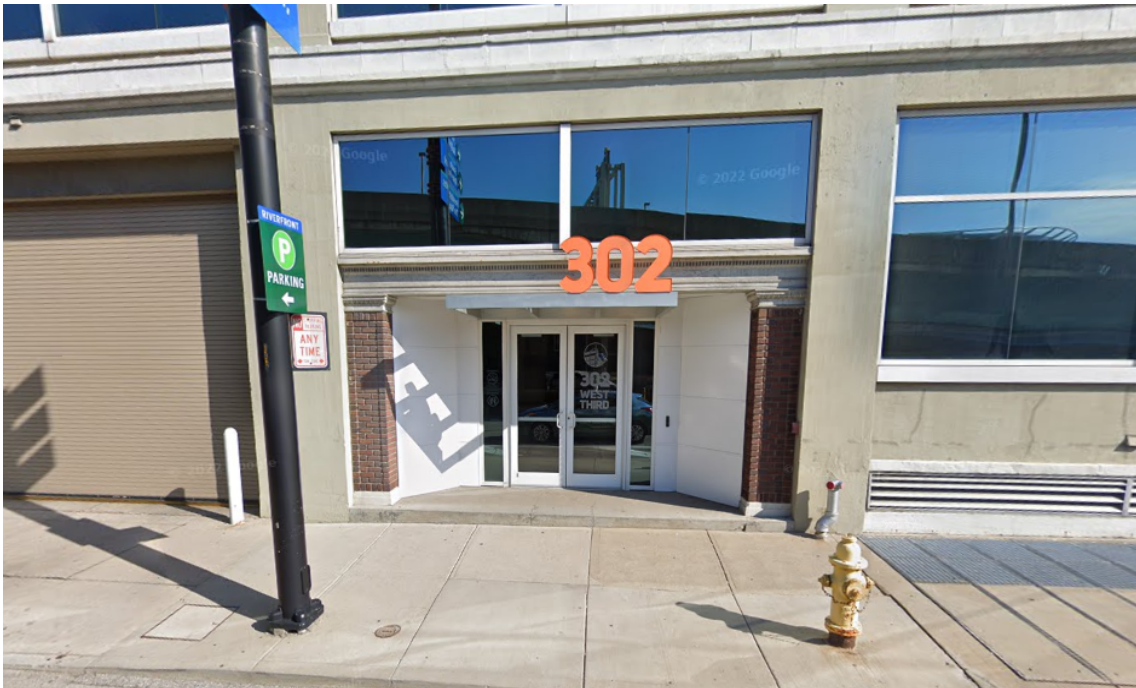
302 W. 3rd Street Entrance
